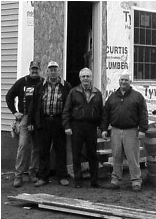
Some of our volunteers from the Glens Falls Building Trades Council take a break at Platt Street. Left to right – Doug Blacklock (Project Foreman), Les Weller, Phil Tucker (President of the Building Trades Council) and Phil Dobie.
